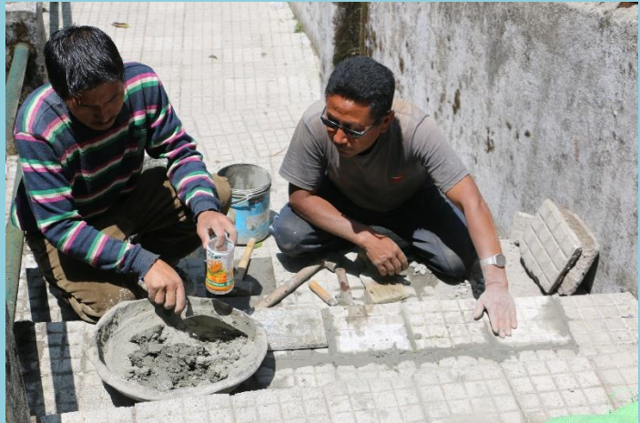
Repair of steps in the visitors pathway
